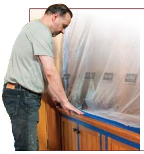
Norton masking tapes feature a special solvent-based, rubber adhesive system and strong holding properties. These tapes adhere and release cleanly while providing clean edges on a variety of flat, contoured, and irregular surfaces. Norton sheetings provides superior solvent, paint, and contaminant penetration resistance. Use them during paint preparation and anywhere you need work area protection. Tear-resistant properties allow movement without ripping.
